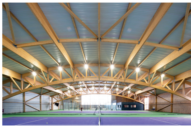
TENNIS & PADEL COUVERT Morainvilliers (78)
