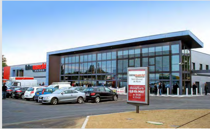
1: Saint-Bonnet-de-Mure (France) Architect: DWA
